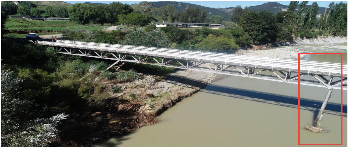
TEPUNA BRIDGE WITH DISCONNECTED PIER OUTLINED IN RED
