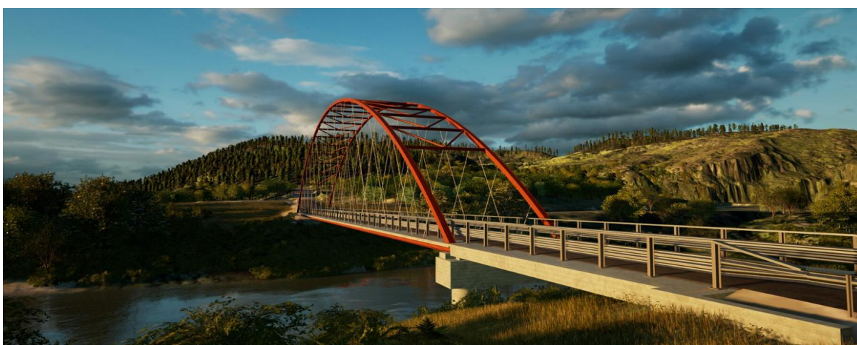
MODEL OF NETWORK ARCH BRIDGE PROPOSED FOR TE REINGA – LOOKING TOWARD RUAKITURI
