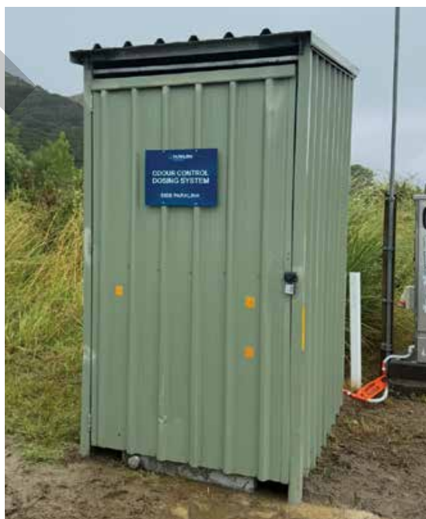
Oputama – odour control, installed December 2024 – doses magnesium hydroxide to help with control odour.
