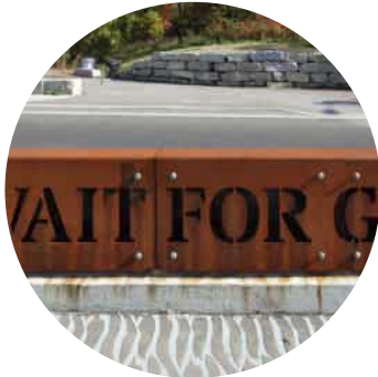
Example of laser cut steel panel fixed to concrete block wall
