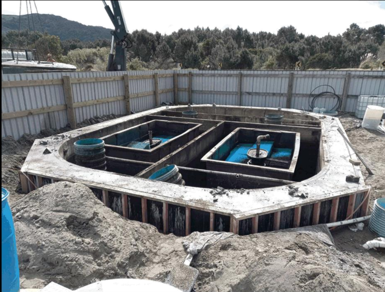
81. Opoutama WWTP - main tank lids removed
