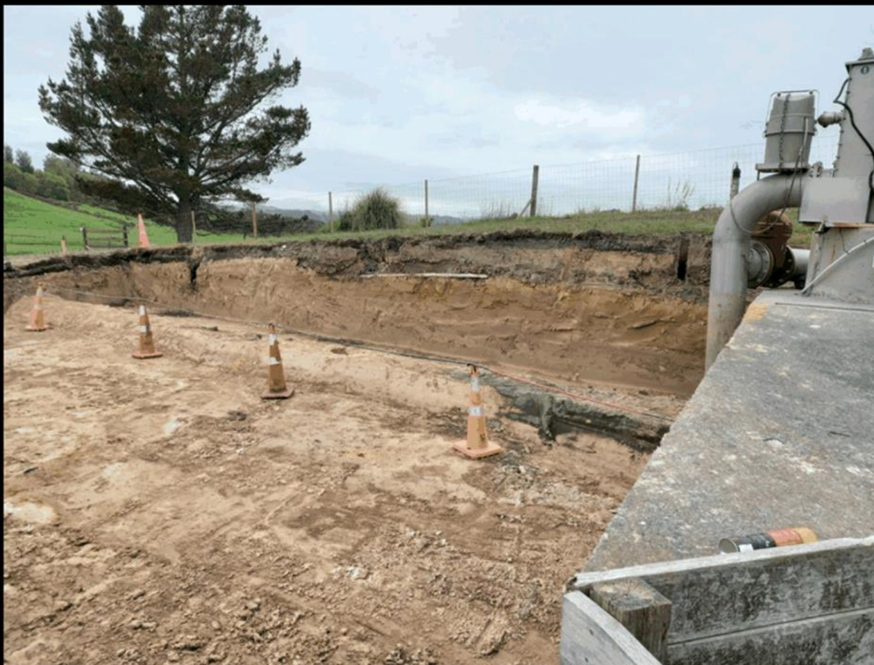
44. Wairoa WWTP - excavation for inlet screen foundation
