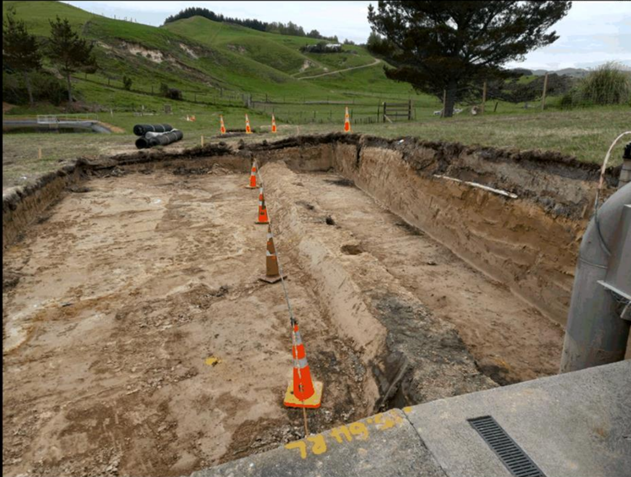
45. Wairoa WWTP - excavation for inlet screen foundation
