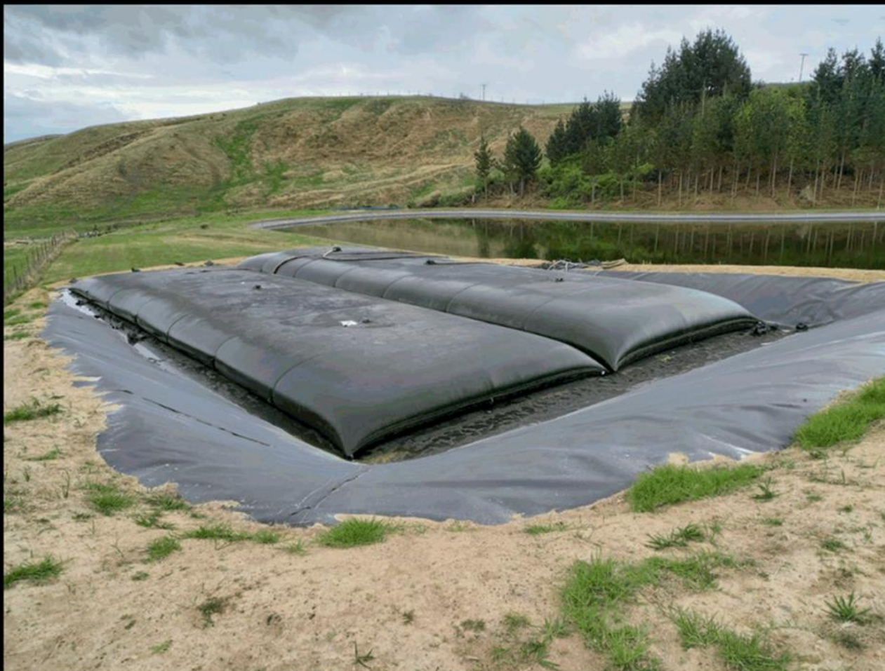
49. Wairoa WWTP - geobag full of sludge for dewatering
