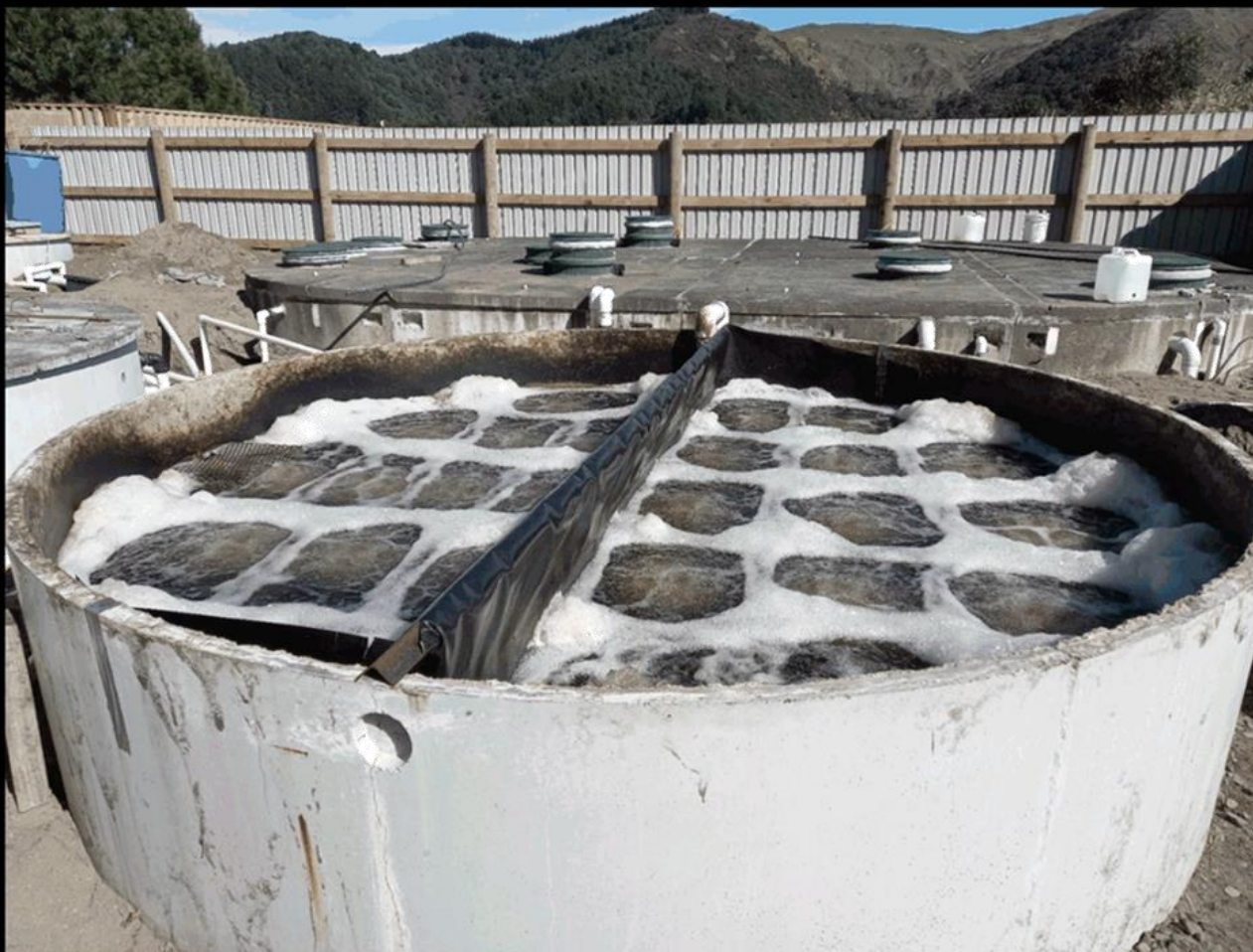
85. Opoutama temp WWTP at 3weeks aerators on
