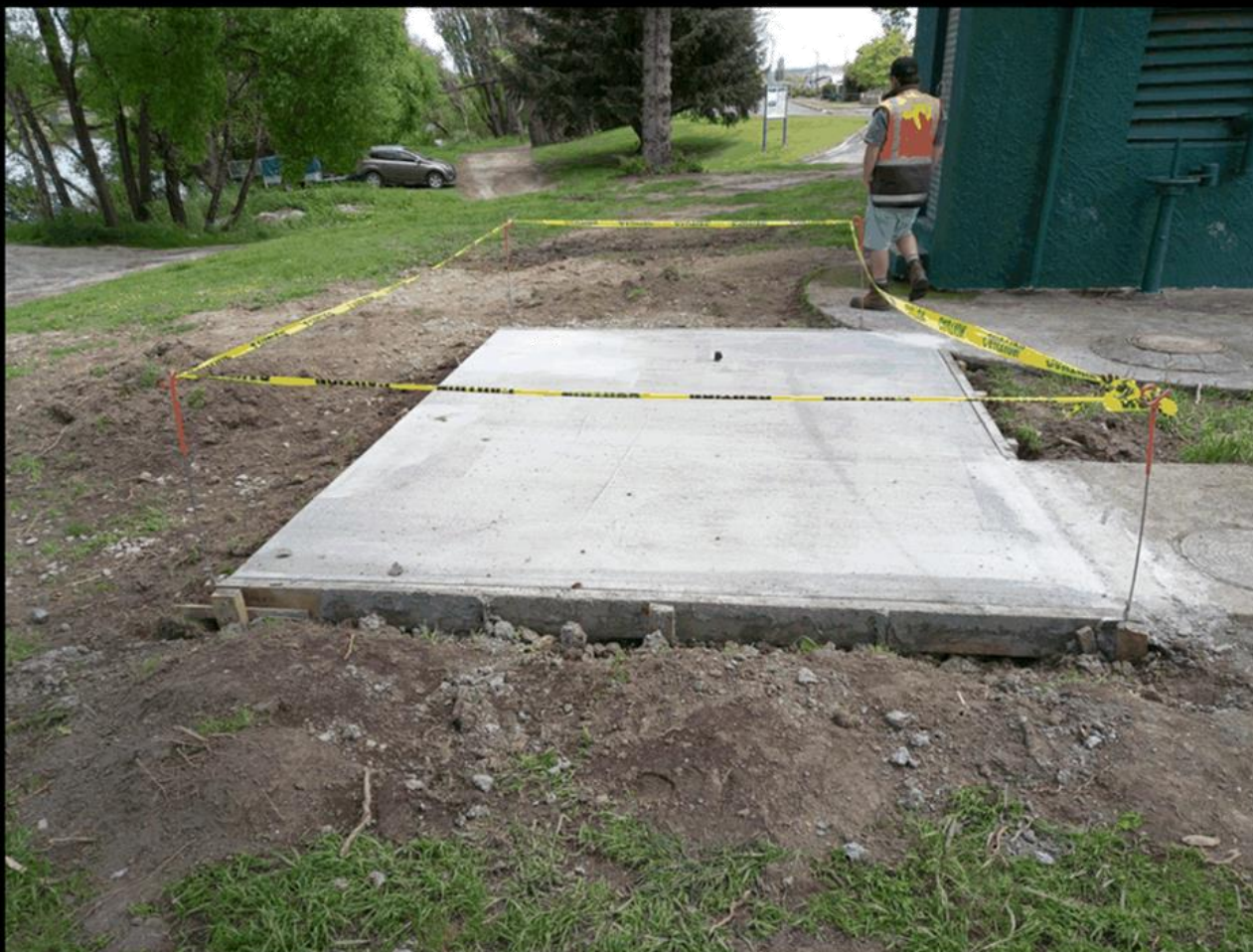
18. WW Pump Station Upgrades - generator pad North Clyde
