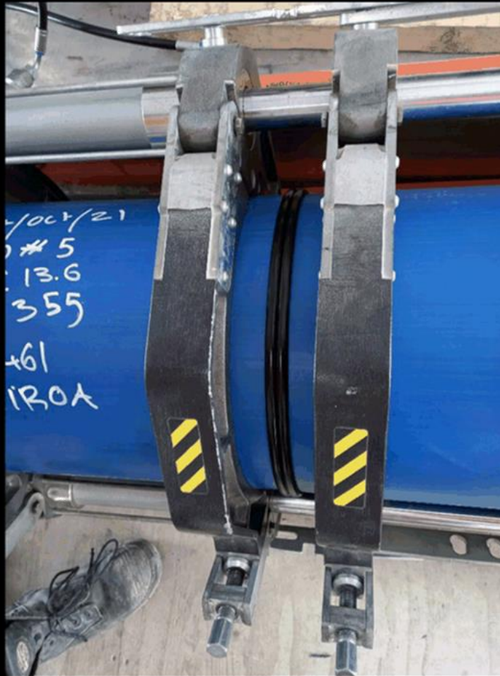
54. Achilles St water main - pipe welding
