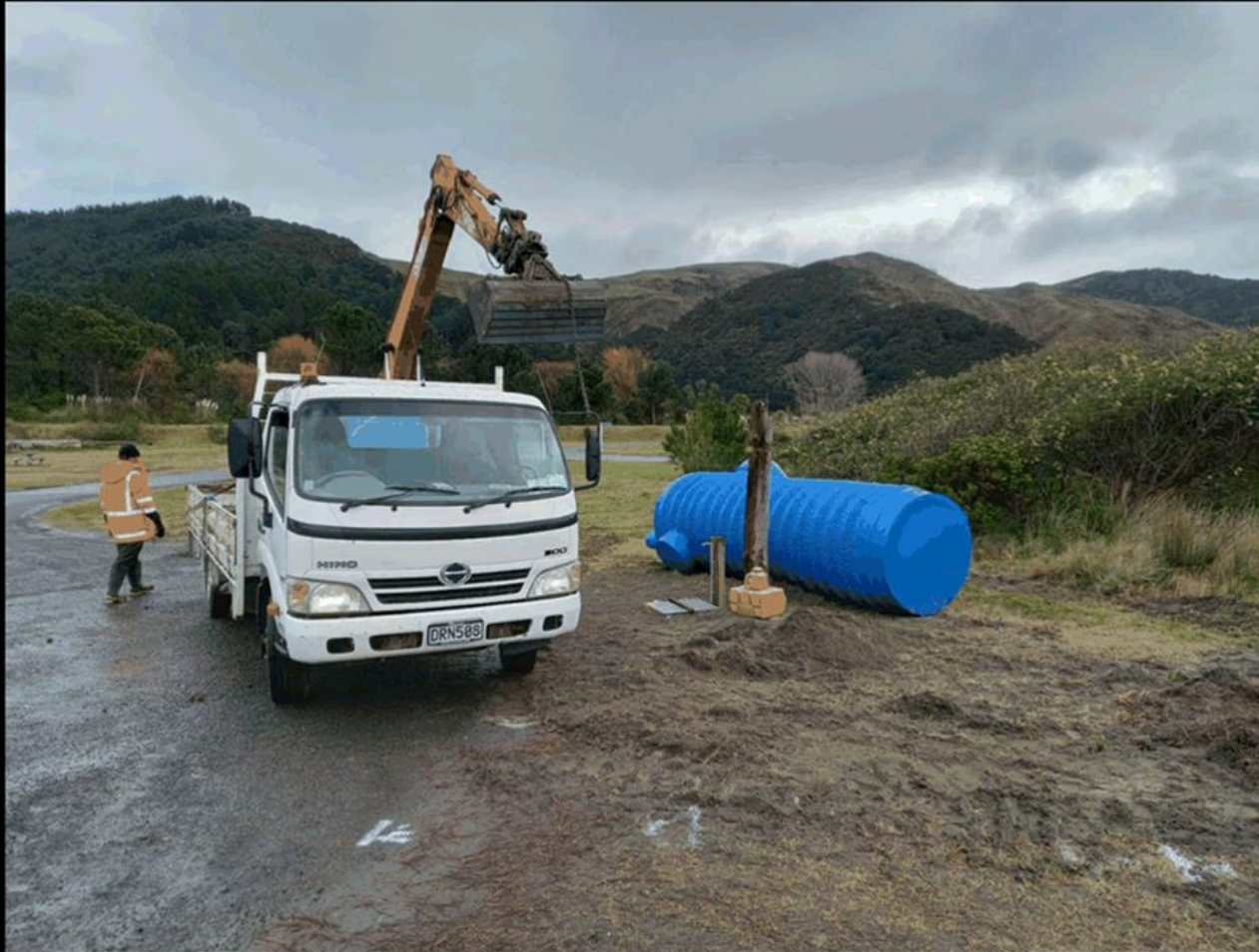
84. Opoutama - Self contained vehicle waste station tanks prior to install
