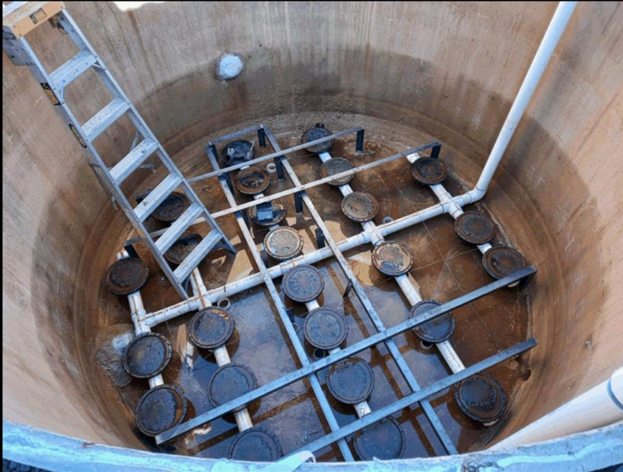
89. Opoutama temporary plant aerators
