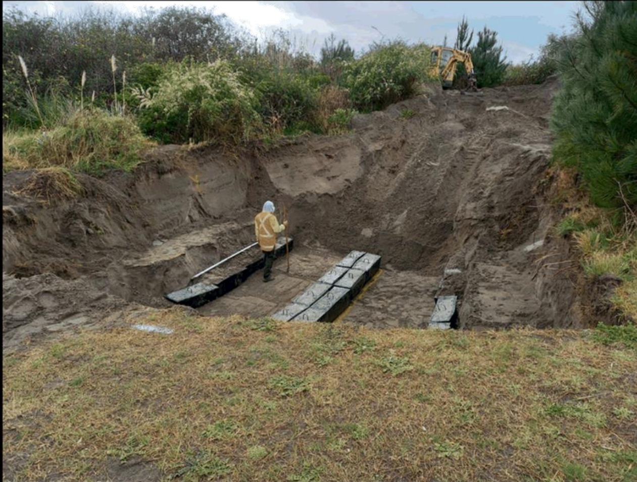
83. Opoutama - Self contained vehicle waste station tanks - digging hole
