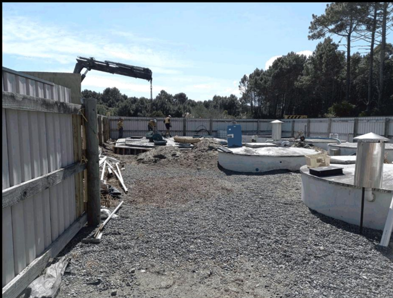
82. Opoutama WWTP - lifting main tank lids
