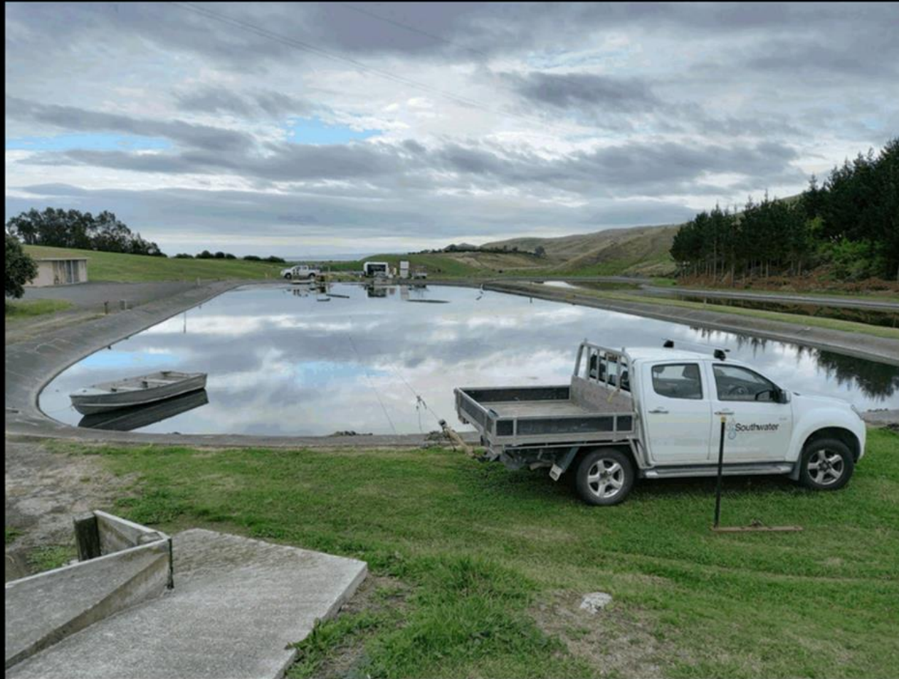
48. Wairoa WWTP - Southwater desludging aeration pond
