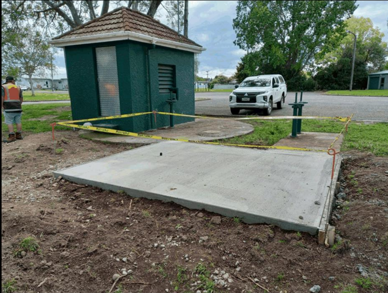
17. WW Pump Station Upgrades - generator pad North Clyde
