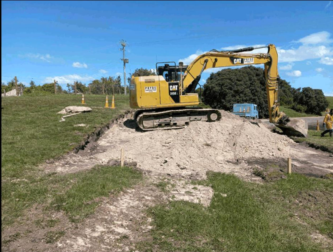
47. Wairoa WWTP - excavation for inlet screen foundation
