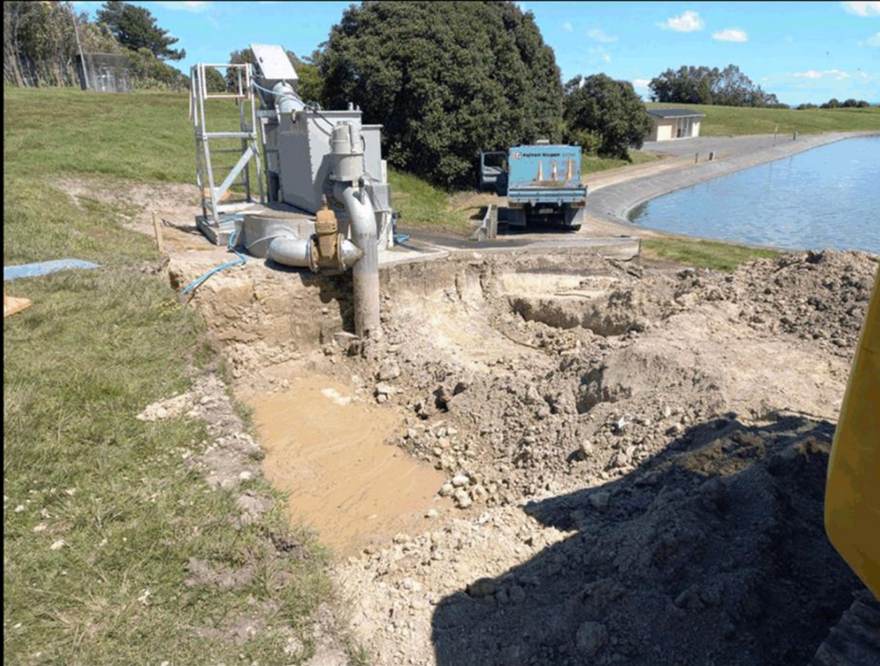
46. Wairoa WWTP - excavation for inlet screen foundation
