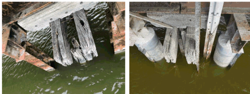
Figure 2 Section loss on web of steel H-Piles
