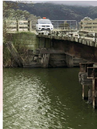
Fig 3: Bridge abutments
