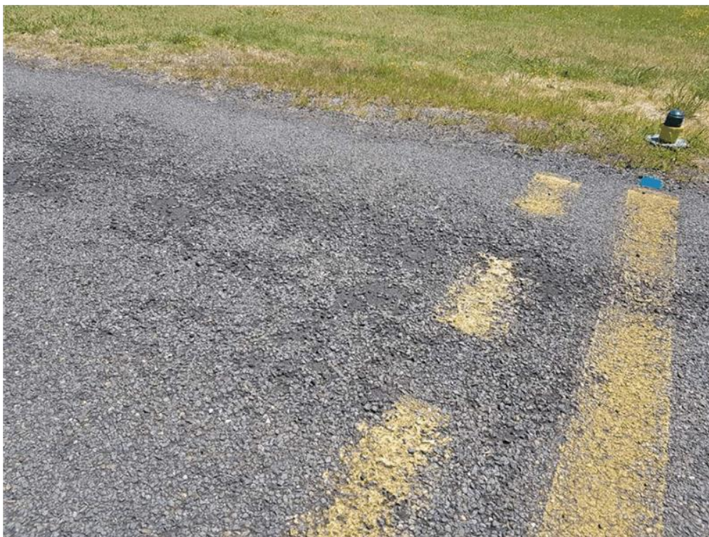
Photo showing chip loss on Taxiway
