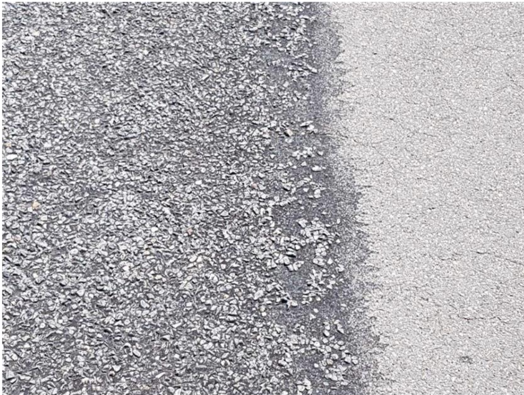
Photo showing Grade 3/5 chipseal and AC surfacing
