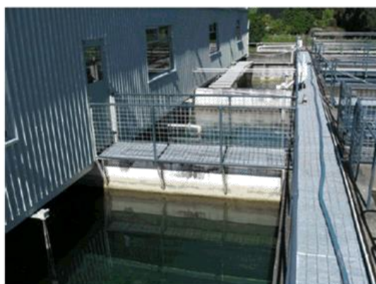
Figure 6 Gravity sand filters
